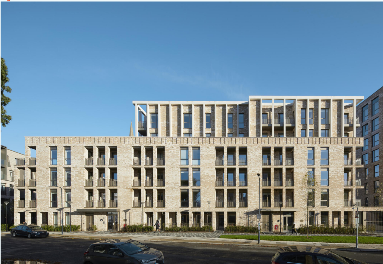
Unity Place by Gort Scott features a well-defined base, middle and top to create an attractive elevation with aligned and regularly spaced fenestration.
