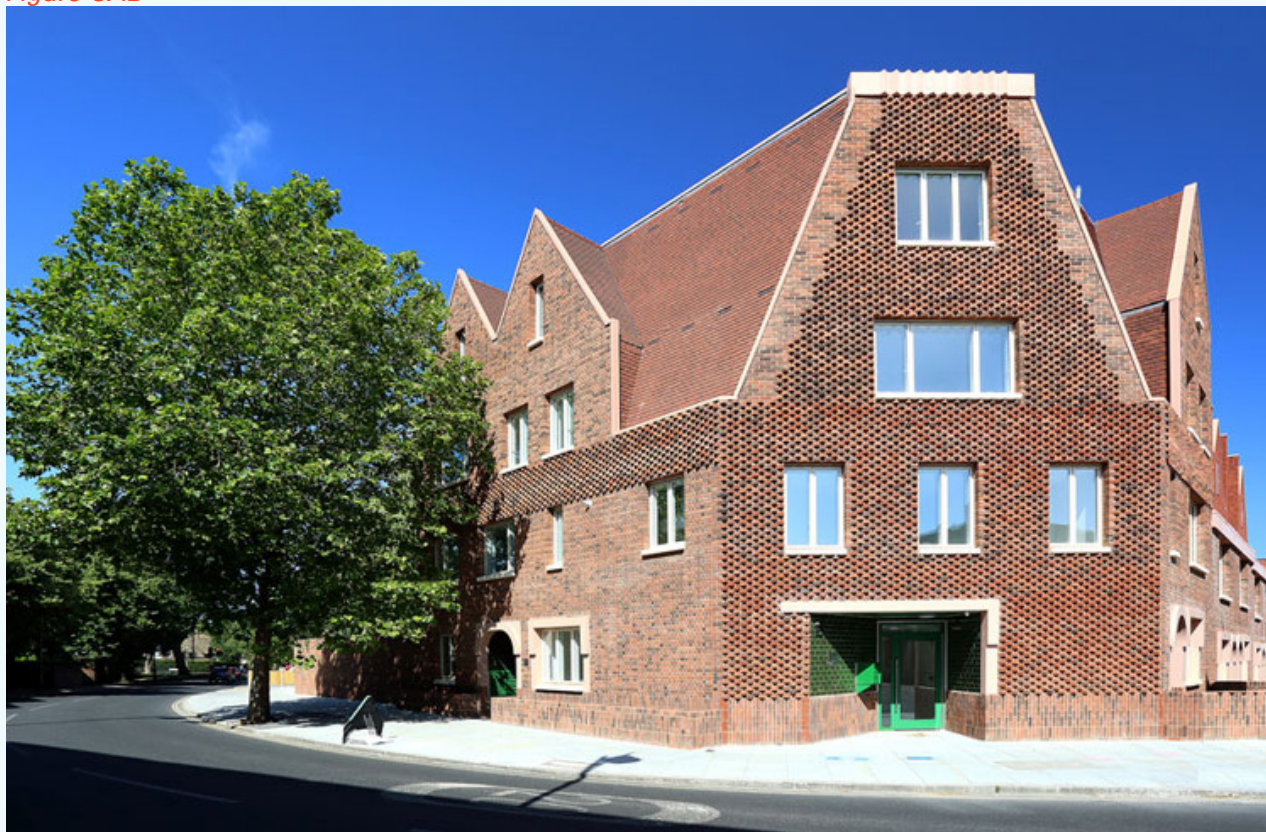
Nunhead Green in Southwark by AOC and David Miller Architects show how roof forms can be used to articulate the top of a four-storey apartment building.
